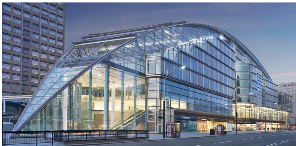
Slika 5. Prikaz objekta izvedenog od stakla tipa SGG COOL-LITE SKN 172 [12] Figure 5. Presentation of the building made of the type of glass SGG COOL-LITE SKN 172 [12]
